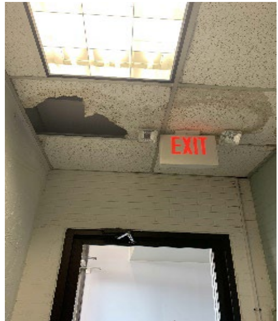
Photograph 2: Water damage
