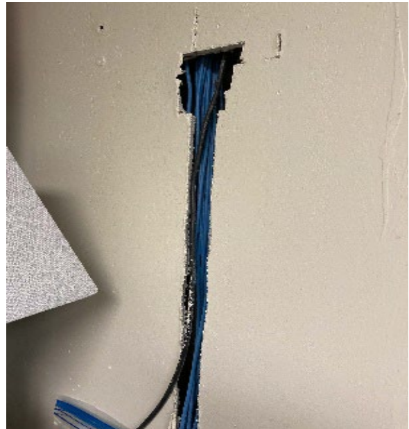
Photograph 4: Exposed wiring
